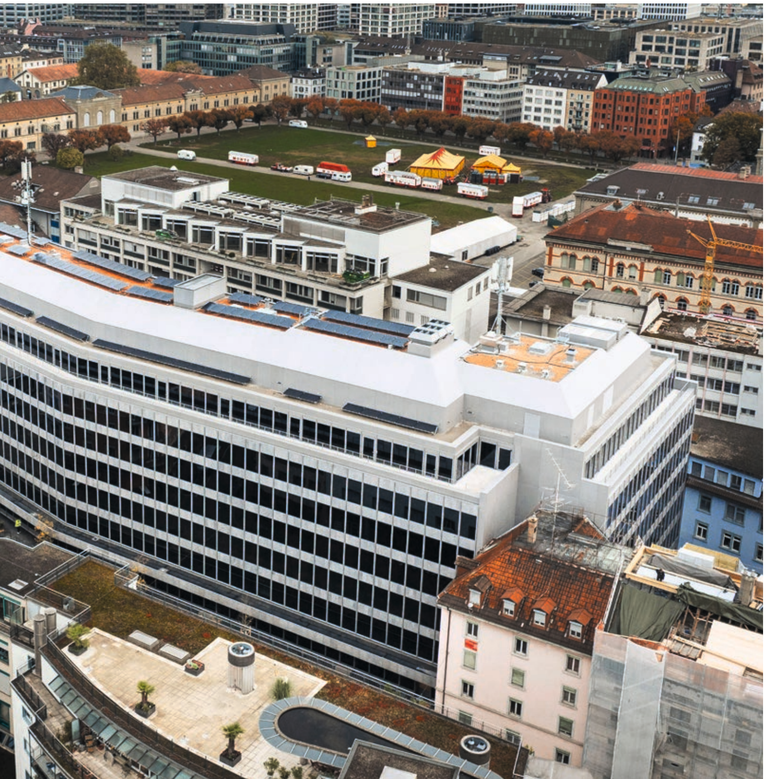
Müllerstrasse is located right by the barracks site in the heart of Zurich city centre.
